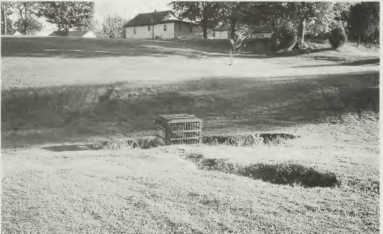
Figure 24 Jerry Lawrence Sink is a large sinkhole that is used to dispose of surface runoff via Streiler City Cave. Water is channeled through exposed segments of the cave ( top photo ) and cascaded down caged entrances ( bottom photo ) to the main part of the cave system. (Stop 6)
